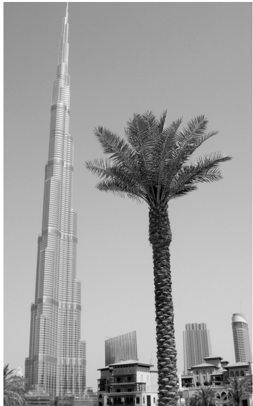
Figure 0.5. The world's tallest building: Burj Khalifa in Dubai.
