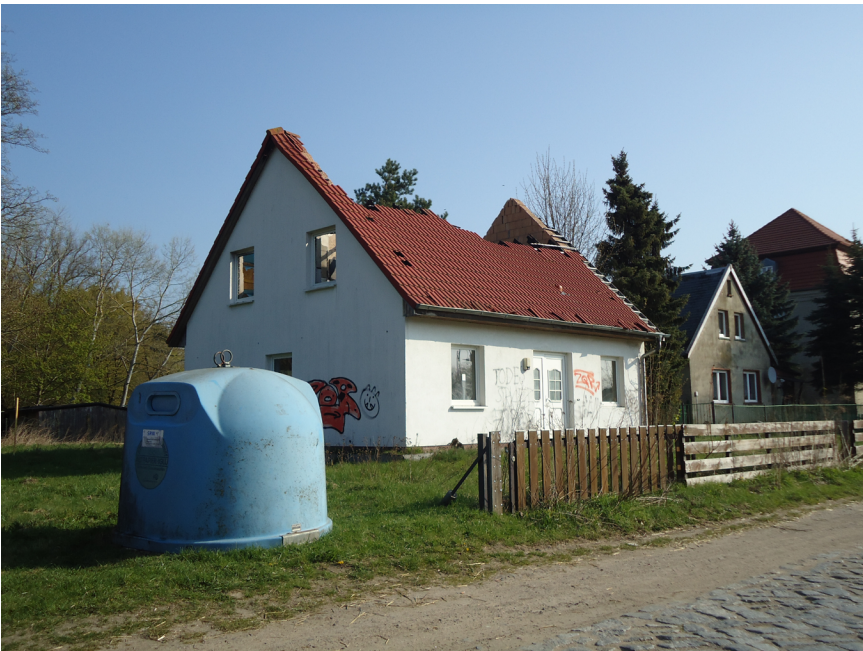
Illustration 1.1. Collapsing House, Mecklenburg-Vorpommern, 2010. Photo: T. Gurr.
