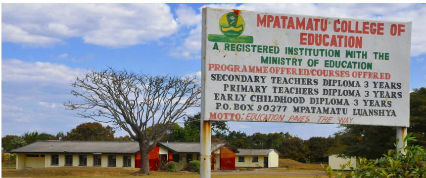
Figure 3.3. Mpatamatu College of Education at former Kabulangeti Community Centre. Photo by the author.
