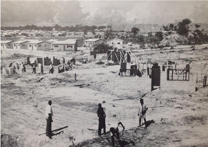
Figure 1.1. Mpatamatu's section 22 under construction, late 1950s. LSE Library Archives, London.
