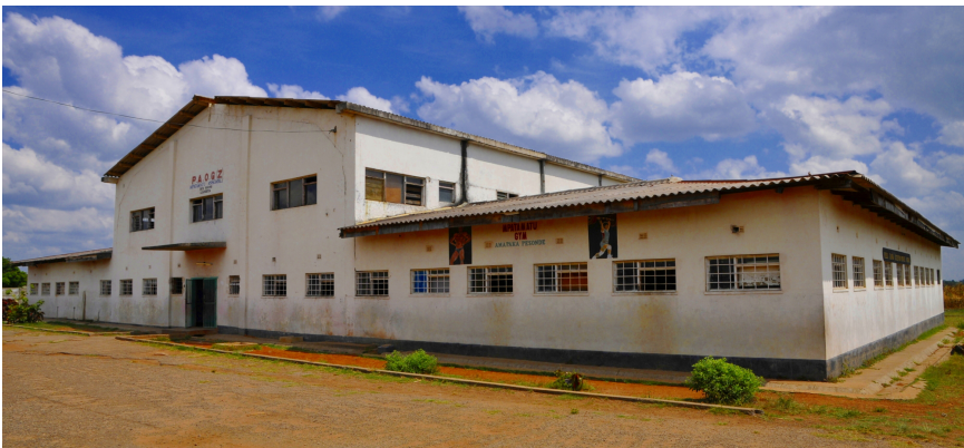
Figure 4.3. Mpatamatu's former sports complex. Photo by the author.
