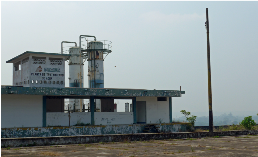
Figure 4.5. Abandoned processing plant at the cuartel in Emiliano Zapata where various decaying industrial installations and provision facilities for company staff are located, Papantla, Mexico, 2016 © Svenja Schöneich.
