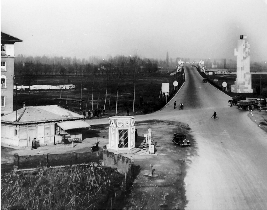
Figure 6.1. Turin, starting point of Turin–Milan motorway, early 1930s. Autostrada Torino–Milano Archive. Courtesy of SATAP, S.p.A.
