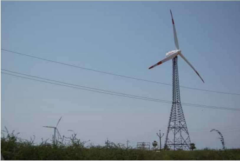
Figure 1.2. Wind turbines outside the nuclear power station in Kudankulam. © Raminder Kaur.
