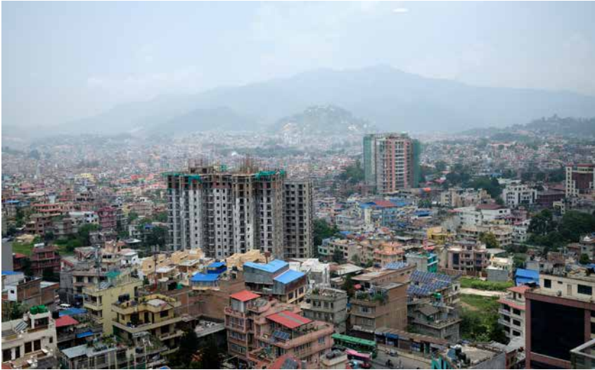
Figure 5.1. Construction site for a luxury hotel in Kathmandu. © Dan Hirslund
