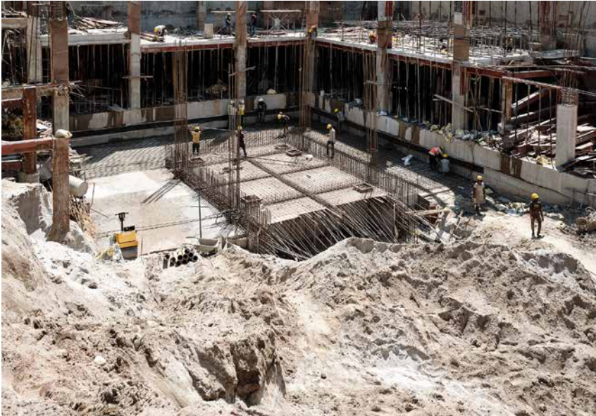
Figure 5.2. Construction of a luxury hotel in Kathmandu. © Dan Hirslund
