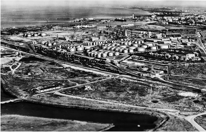
Figure 10.1. The Dunkirk refinery with the Cité des Ingénieurs, France. Photo: © CMUA-Archives de Dunkerque (fonds SRD), used with permission
