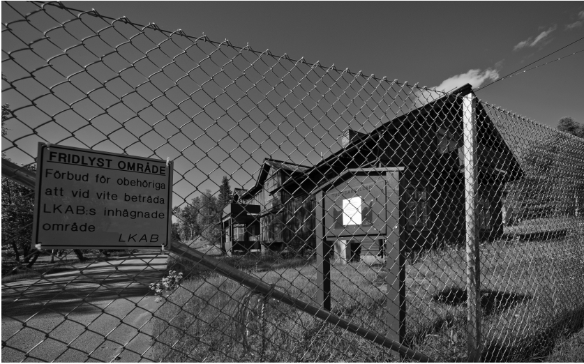
Figure 5.2. One of the historic buildings in Malmberget, behind the enclosure. Photo: Daryoush Tahmasebi © Norrbotten's Museum
