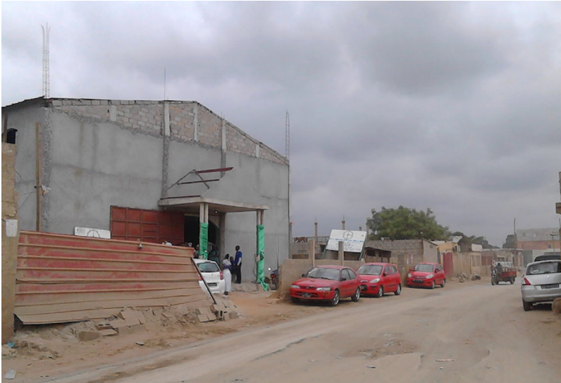
Figure 3.3 Christian church under construction in Sapu, Luanda. Photo by Ruy Llera Blanes.
